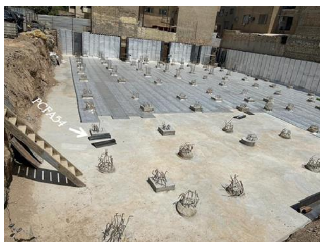
Figure 2. Testing pile PCFA54 installed with CFA method
