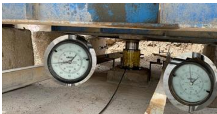
Figure 4. Dial gauges' readings during 150 Tons load test
