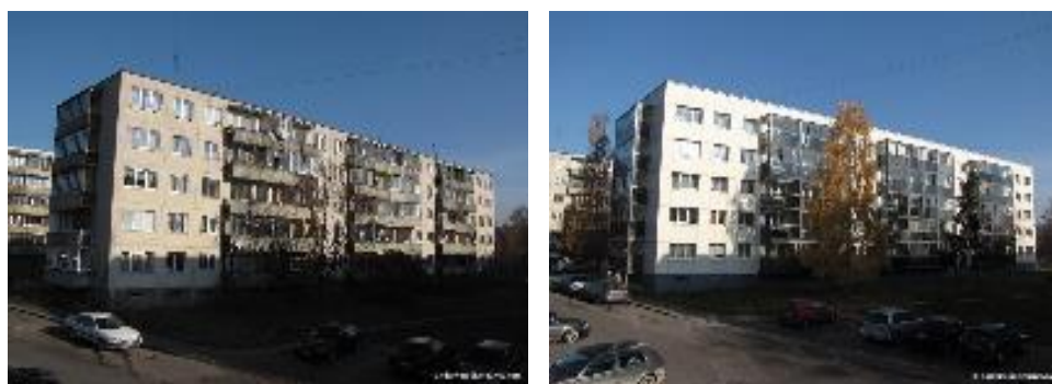
Figure 6. The result of reconstruction of a typical panel house of series 1-464 in the district of Zhirmunai, Vilnius, Lithuania
