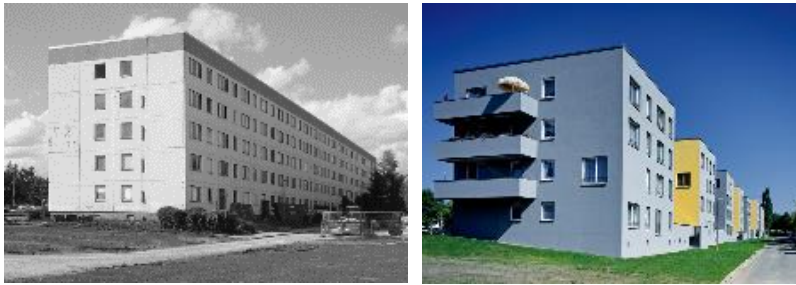
Figure 2. The result of the reconstruction of panelized housing designed by Stefan Forster Architects, Linefelde, Germany
