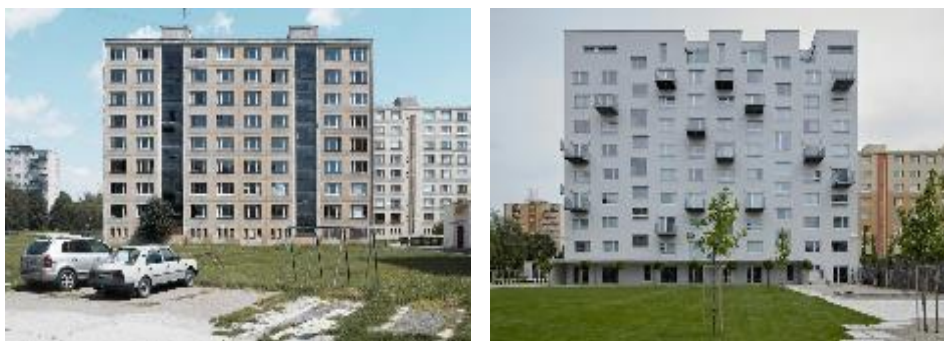
Figure 7. Result of the facade reconstruction of a panel house in Rimavská Sobota, Slovakia
