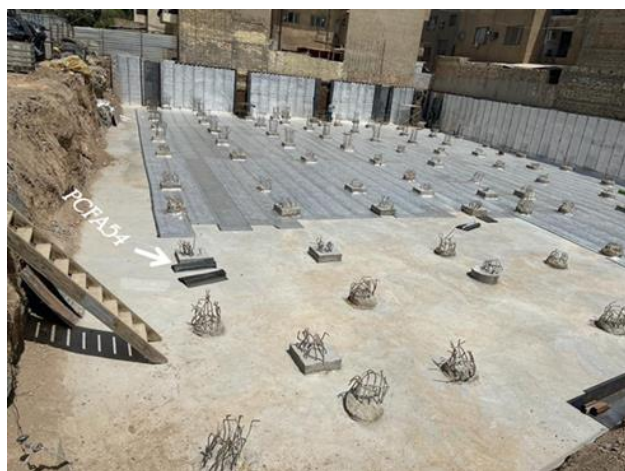
Figure 2. Testing pile PCFA54 installed with CFA method
