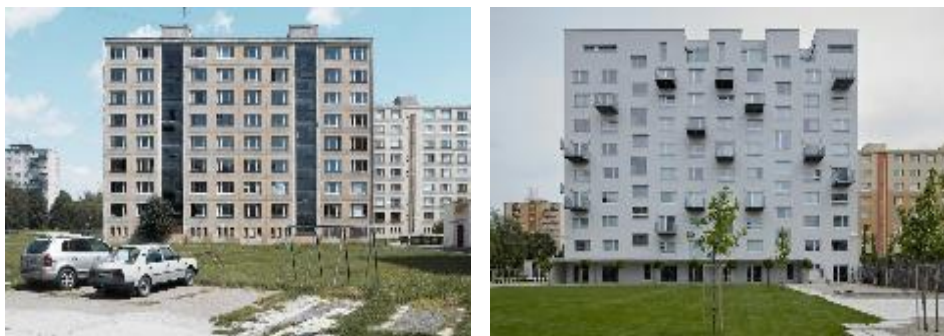
Figure 7. Result of the facade reconstruction of a panel house in Rimavská Sobota, Slovakia
