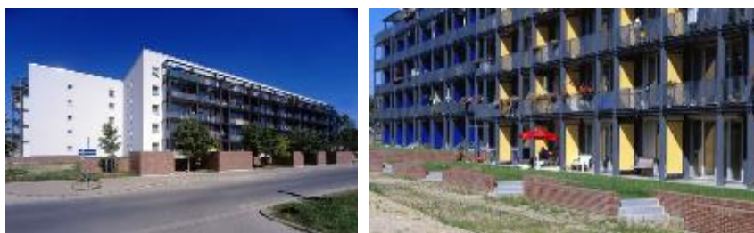
Figure 4. Improvement of panel housing, Linefelde, Germany.
