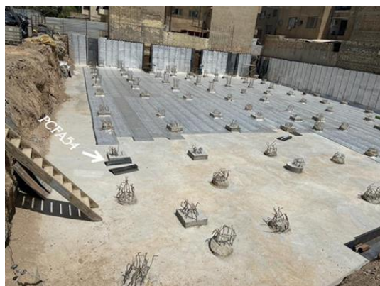
Figure 2. Testing pile PCFA54 installed with CFA method
